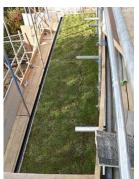
Green roof holds a large amount of water attenuates flow off site
